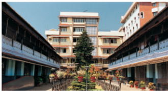
Ayurvedic Hospital & Research Centre, Kottakkal (Tel. No. 0483 2808000)
